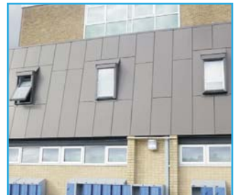
Rockpanel External cladding board manufactured from sustainable rock fibre.
