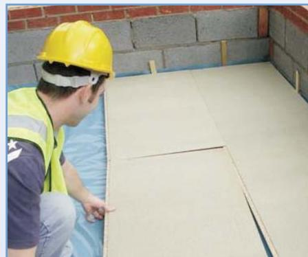
All joints should be bonded using Water Resistant PVA Adhesive. Each board should be tamped with a suitable block, tight-up against the adjoining board.
