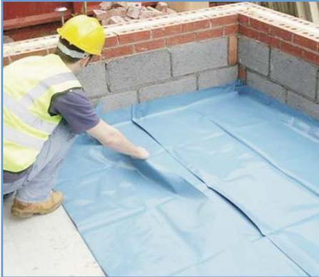
On new floors, the use of a floor screed, is not required, providing that the floor is level and reasonably tamped down. The incorporation of a damp proof membrane should be in accordance with the BS Code of Practice 102: 1973.
